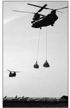
A CH-47 Chinook from the Oklahoma National Guard prepares to place two 7,000 pound sandbags in one of the New Orleans levee breaches.
