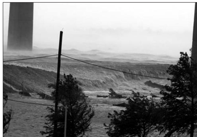
The storm surge from Hurricane Katrina overflows the north levee of the Mississippi River Gulf Outlet/Intracoastal Canal.
